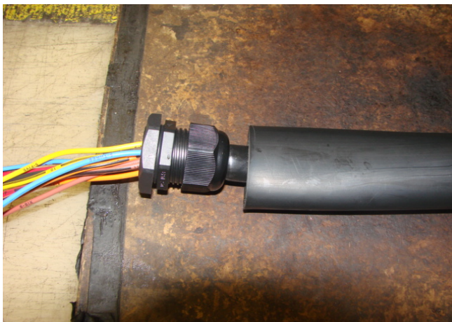
Shrink tube installed onto flat cable boot
